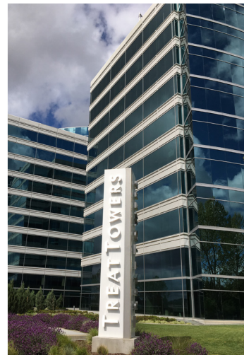
Lack of local control in Orinda could mean the construction of high-rise, high-density buildings in the city.
